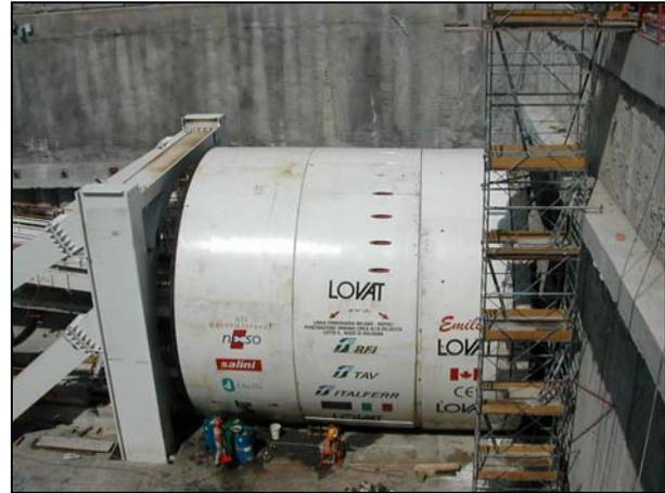
Figure 7 – EPB machine at start-up
