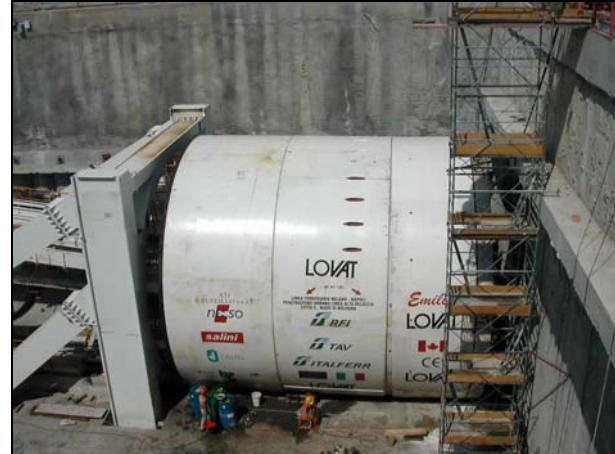
Figure 7 – EPB machine at start-up
