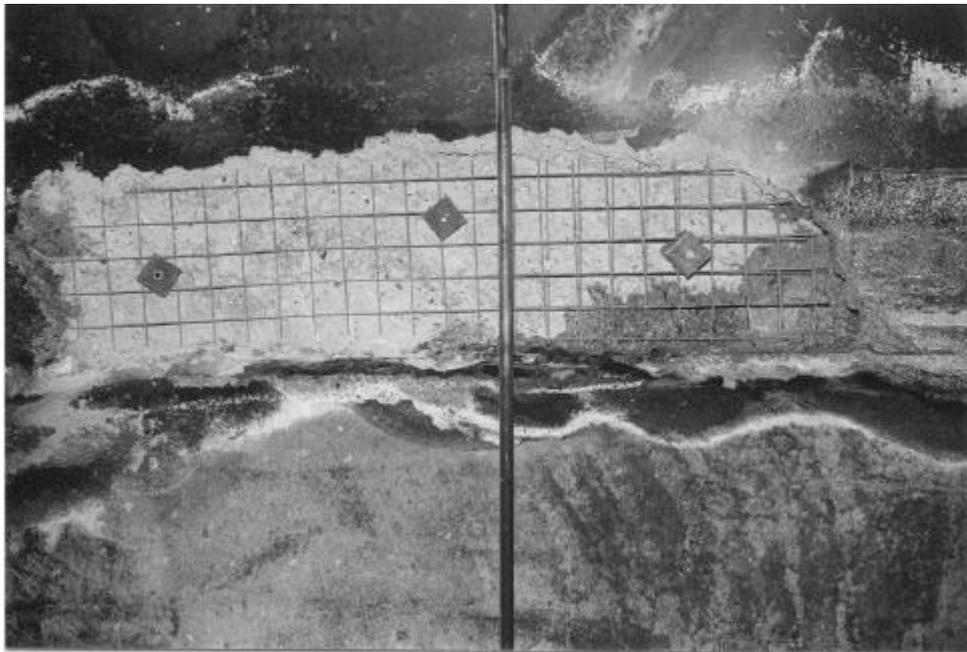
**Figure 2** - Honeycombed concrete demolished and reconstructed using welded wire mesh and dry-mix shotcrete
