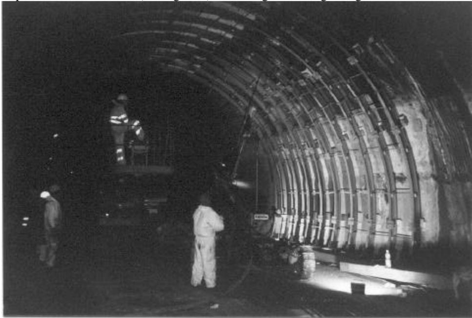
**Figure 4** – Rock bolt installation under protective steel ribs
