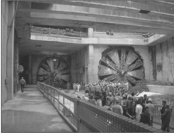
Figure 4. EPB's breakthrough
