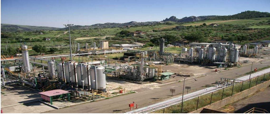
Figure 1. Landscape with the gas power plant
