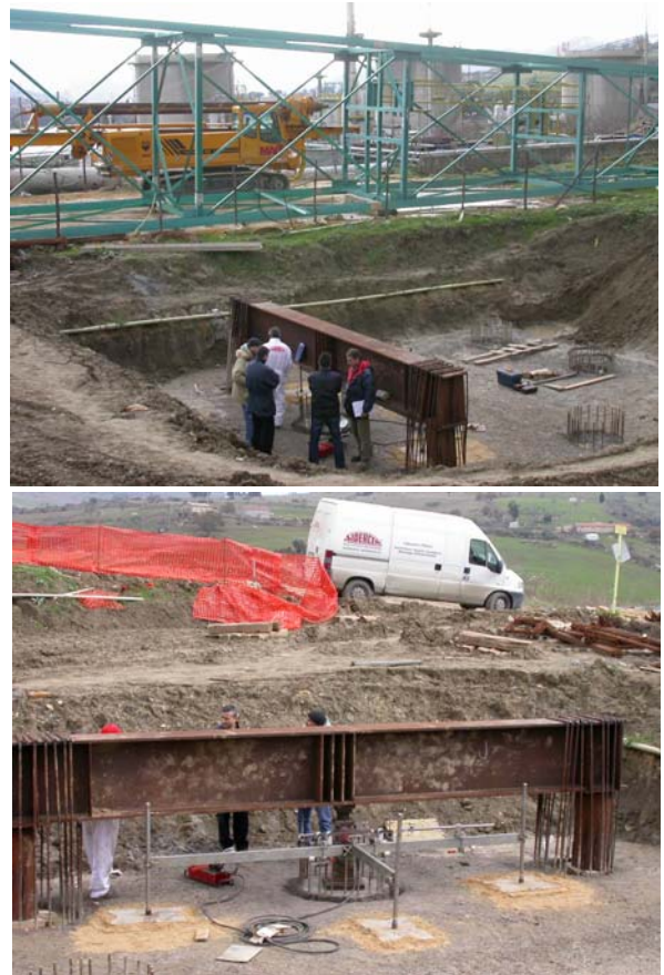
Figures 6. Loading test on pile # 5 of the blow-down system.
